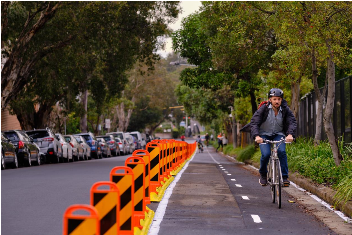
Figure 5: City of Sydney tactical cycleway along Henderson Road, Eveleigh
