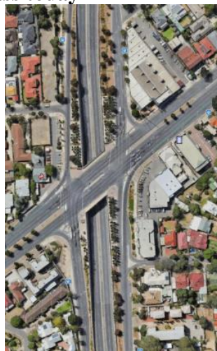
369 Figure 12 – South Road underpass today
