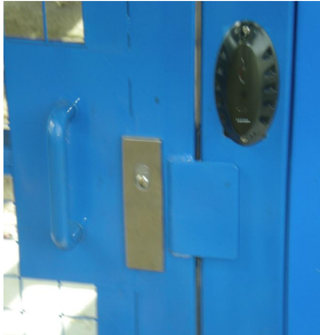
Figure 6 – Parkiteer cage door lock and proximity card reader
