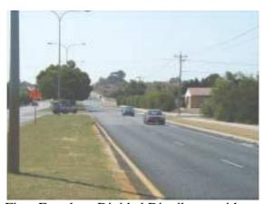
Figure Five: Four lane Divided Distributor without driveway access
